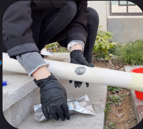
Apply Epoxy Putty
