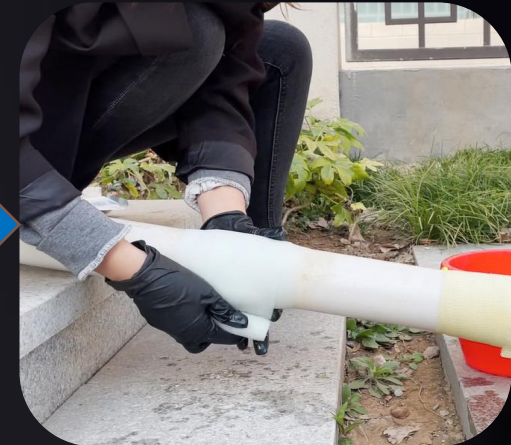
Wrap Spirally and Firmly
